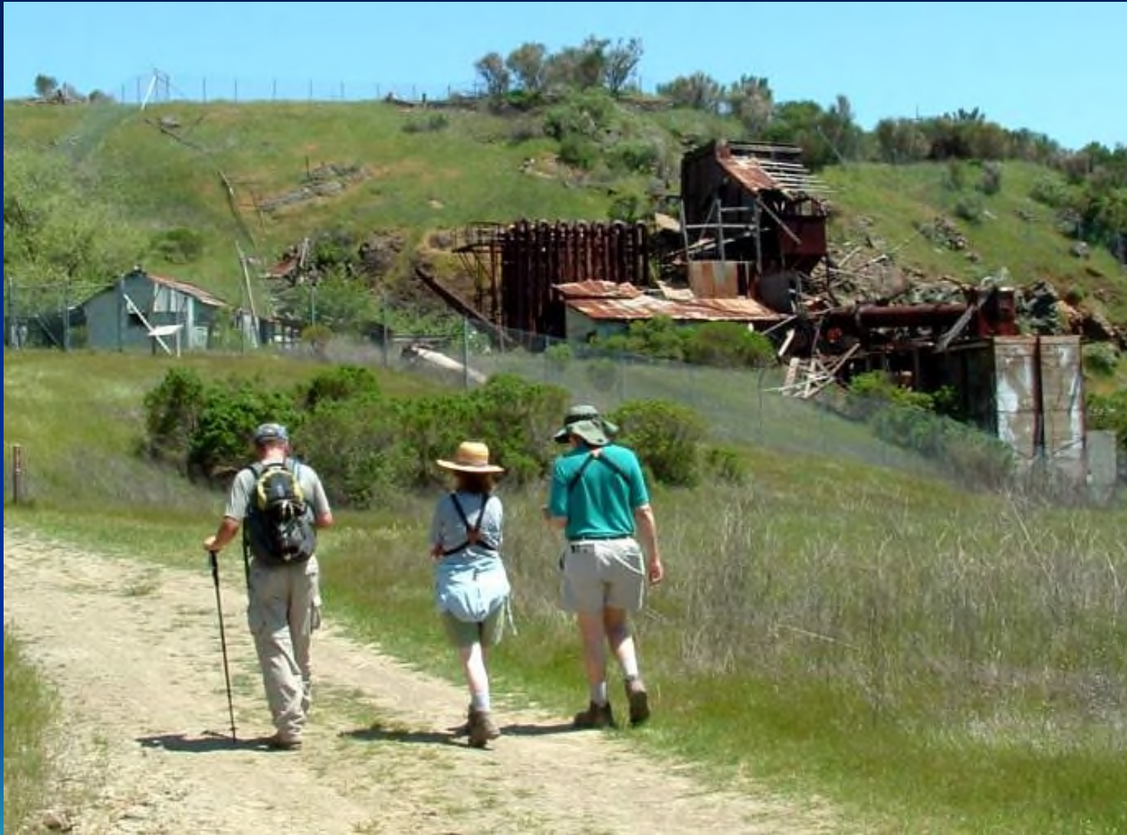
Mine Hill Rotary Furnace, Almaden Quicksilver County Park
